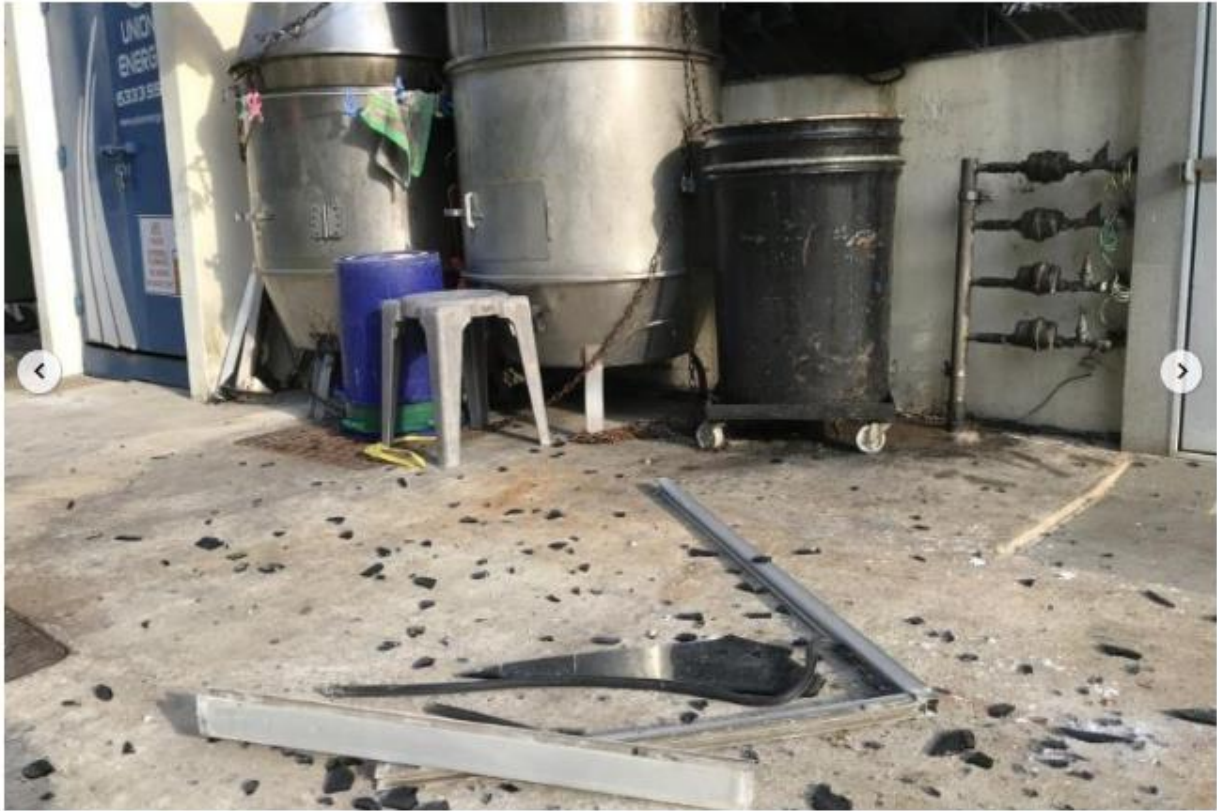
1 of 2 The window panel hit the ground behind a coffee shop at Block 116 Lorong 2 Toa Payoh on Nov 19, 2018. PHOTO: LIANHE WANBAO
