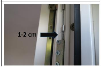
Now fix the second plate using the screws recommended by the window profile supplier or manufacturer.
