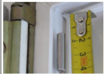
After fixing the first perforated plate, pull the cable to fix the second perforated plate onta the sash.
