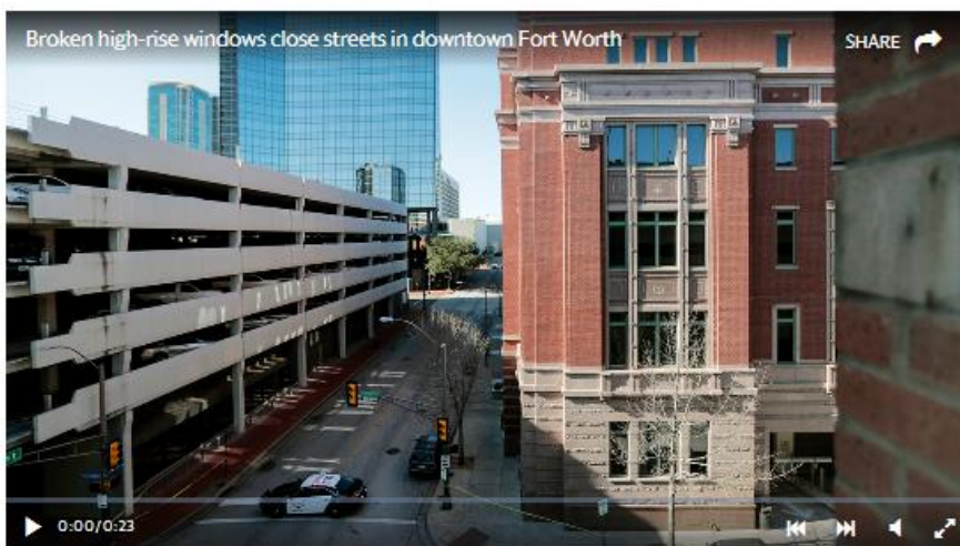
A cable from a window washing apparatus broke out windows on the 17th floor of the Wells Fargo Tower in downtown Fort Worth. Streets surrounding the building were closed Tuesday morning. No injuries were reported. BY AMANDA MCCOY
