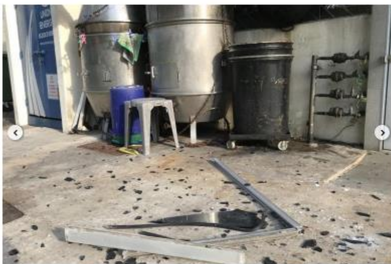
1 of 2 The window panel hit the ground behind a coffee shop at Block 116 Lorong 2 Toa Payoh on Nov 19, 2018. PHOTO: LIANHE WANBAO
