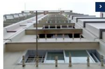
Related Story 50 cases of falling windows in 2017 - a five-year high
